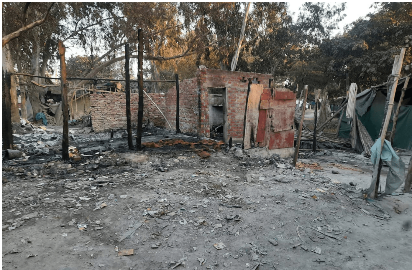
Destroyed houses at Shakur Basti, New Delhi November 2023, Credits: HLRN
