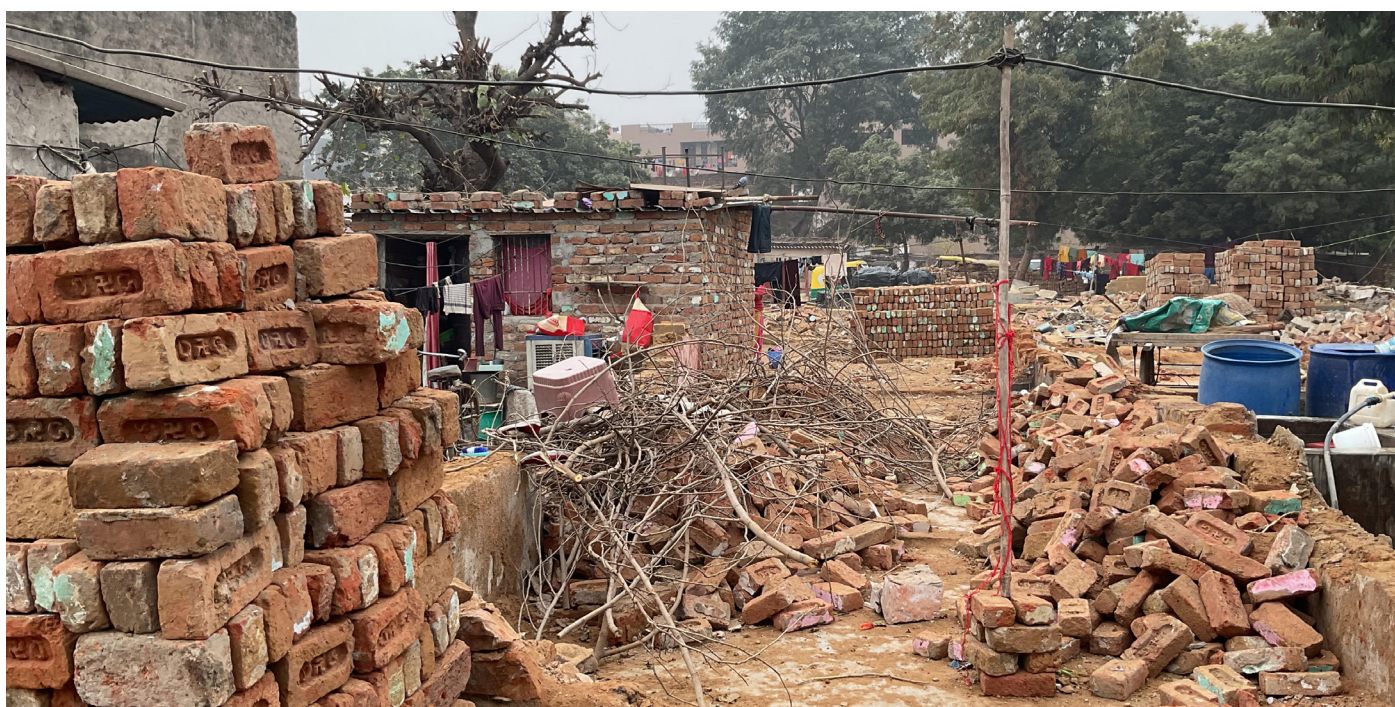
Demolished Houses in Kanhaiya Gaon, Gurugram, Credits: HLRN
